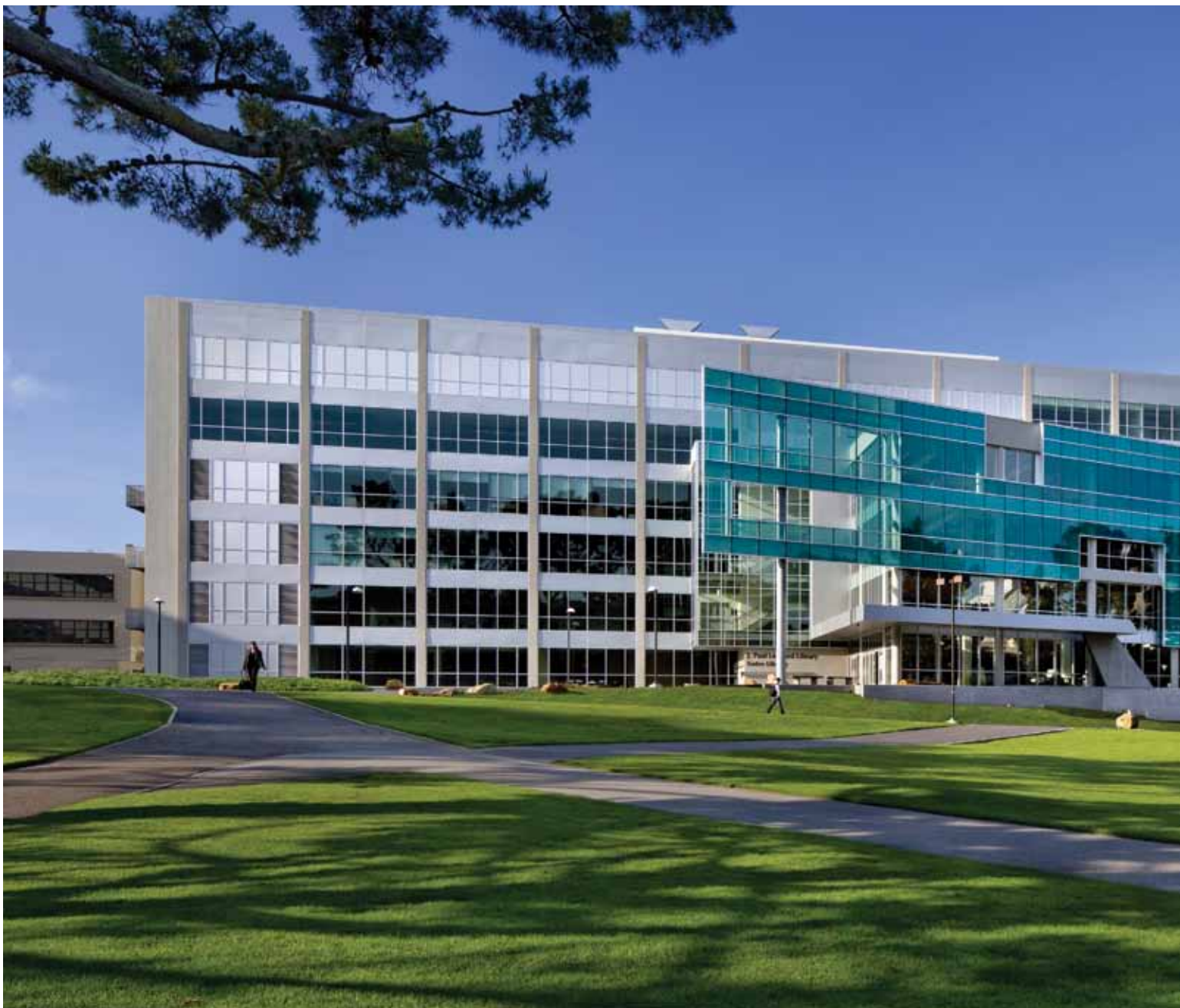
The sparkling glass and steel front façade of the new Sutro Library and J. Paul Leonard Library provide an inviting entrance from the Quad of San Francisco State University. The Sutro Library is on the fifth and sixth floors. Courtesy HMC Architects.
