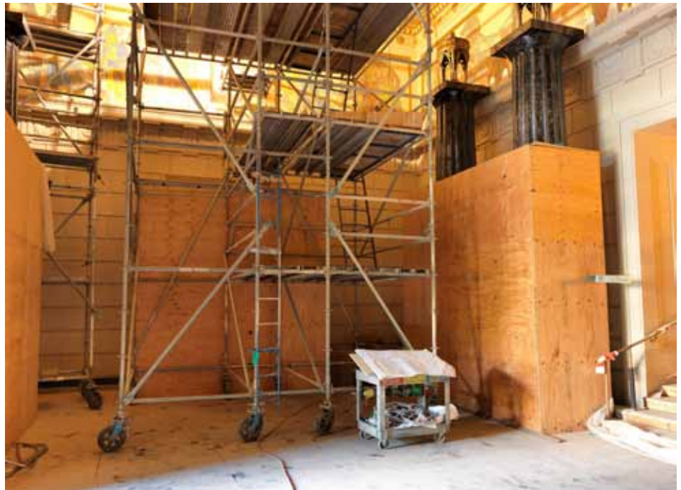
Documented in this photograph is an example of the extraordinary protection given to the decorative elements in the Memorial Vestibule. Photography by Vincent Beiderbecke
