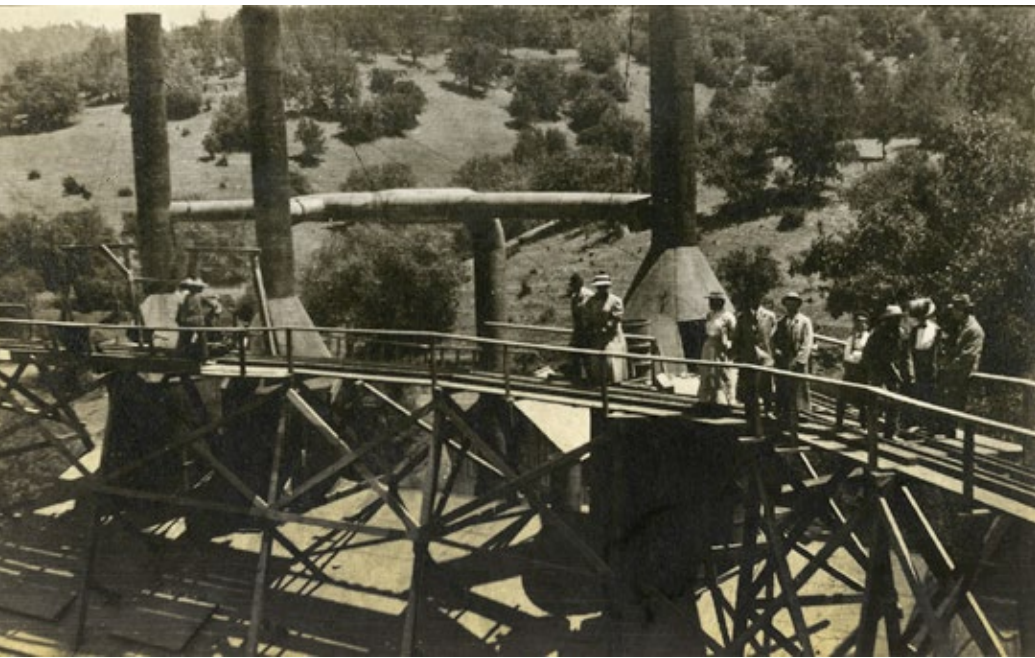
The same party of Sacramento visitors stand on part of the later limekiln furnaces used for processing the limestone quarried at the Alabaster mine.
