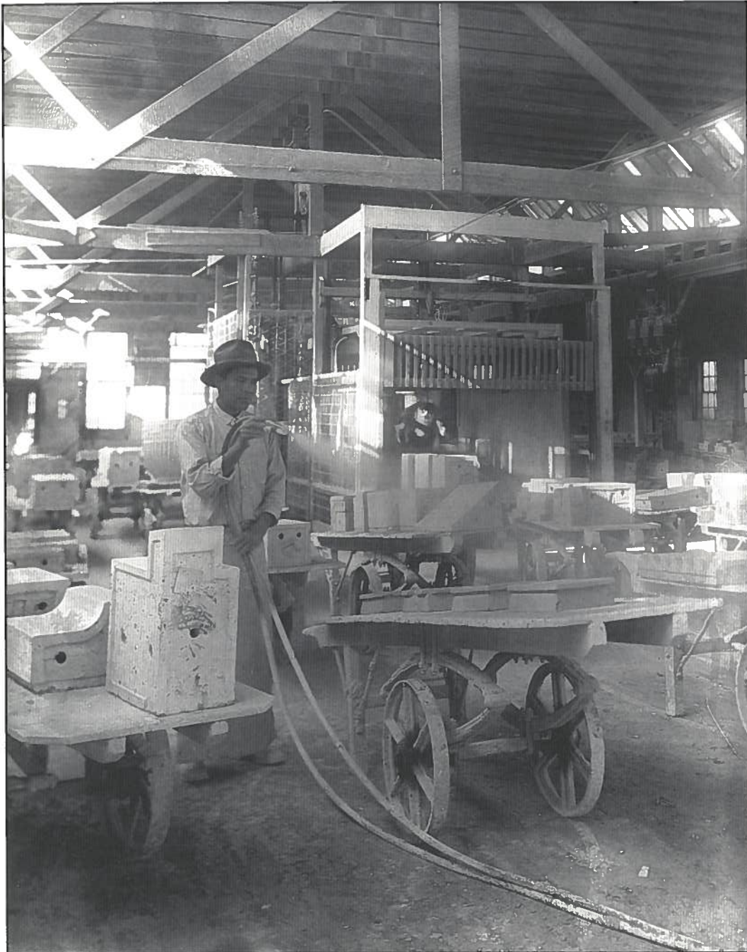
Worker spraying glaze on terra cotta at the Lincoln plant.
