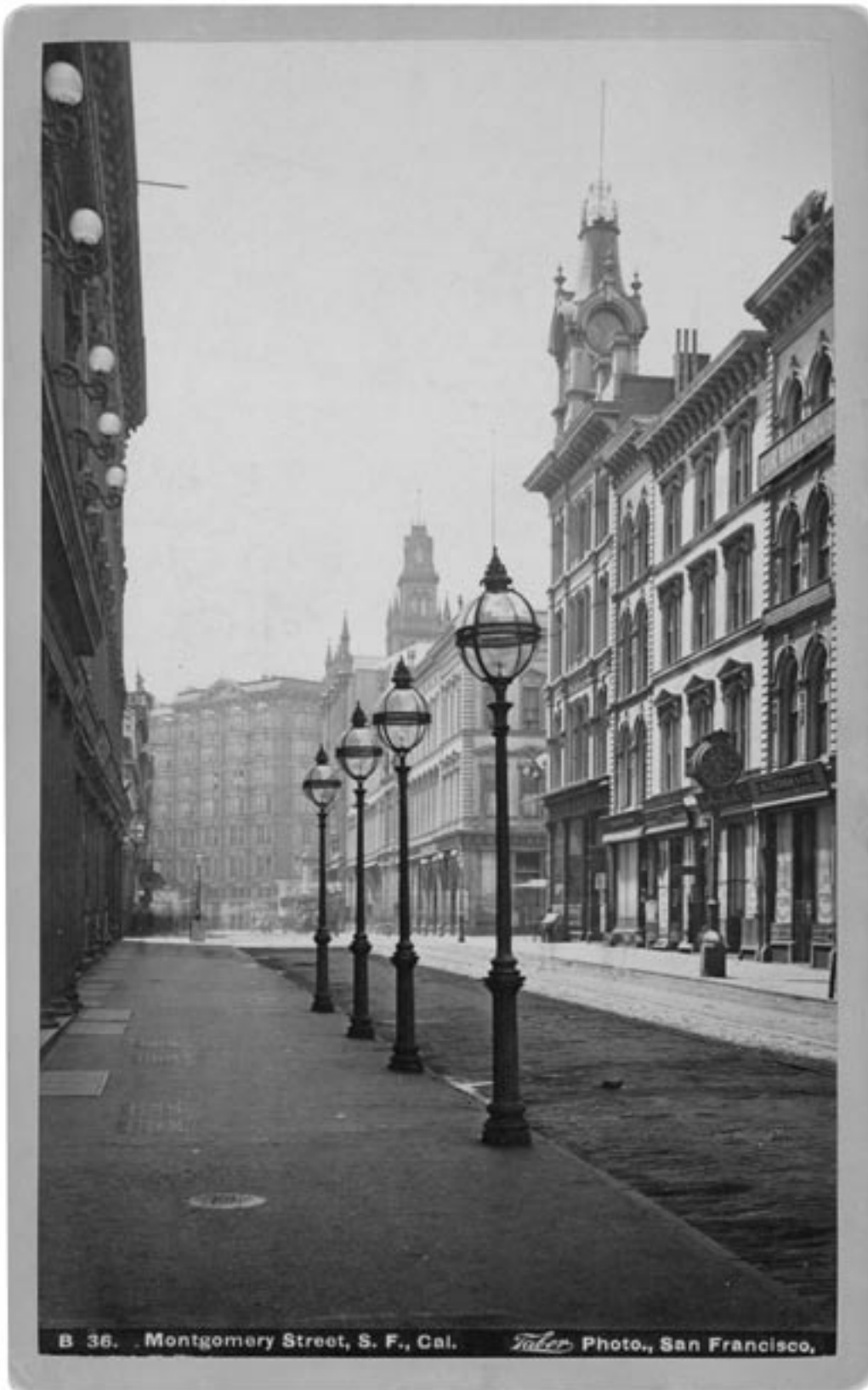
Looking down San Francisco's Montgomery Street with the Palace Hotel in the background.
